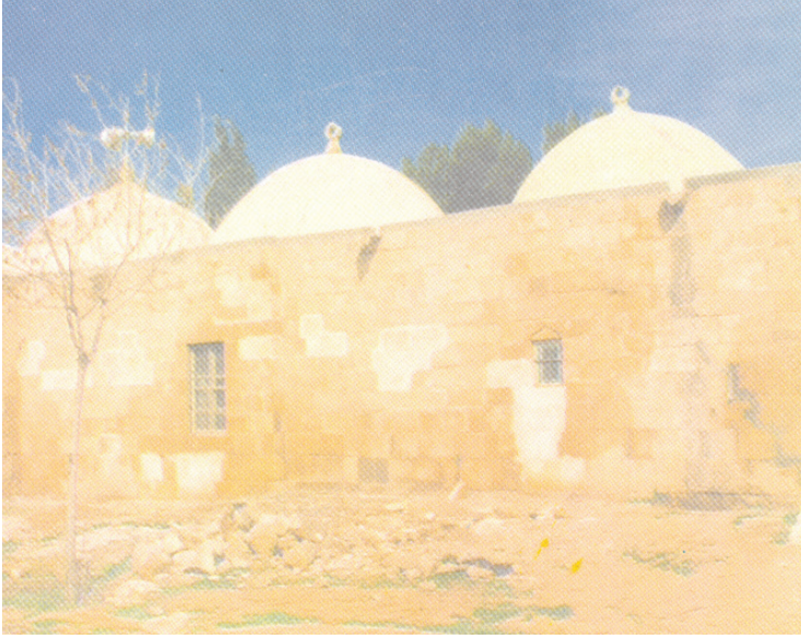
Cabir el-Ensar Camii
